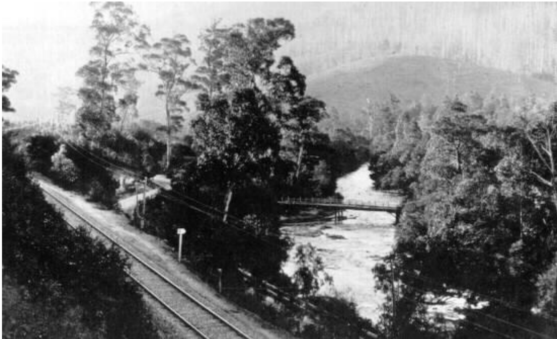
Warburton Railway line and Damman Bridge (printed: Warburton Ways - E. Parkinson)
